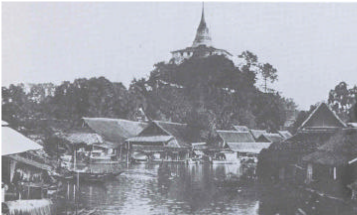
The 'Golden Mount': the manmade, sixty-four metres high, brick edifice, completed in 1878 and camouflaged to pass as a real hill rising from the dead level of the delta, even planted with trees to sustain the illusion. Source: Campbell, J.G. D., Siam in the Twentieth Century London, 1904.
